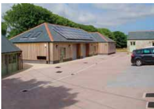
Providing a modern, rural workspace
